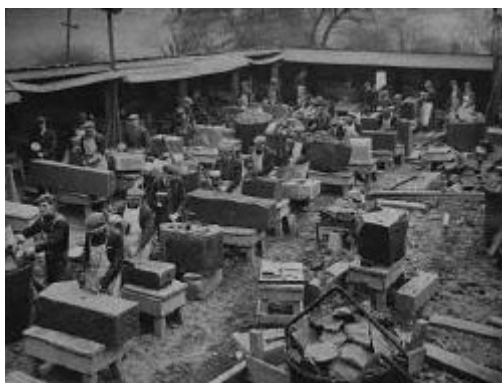
Stone masons repairing the Liverpool Cathedral after its bombing during World War II.
